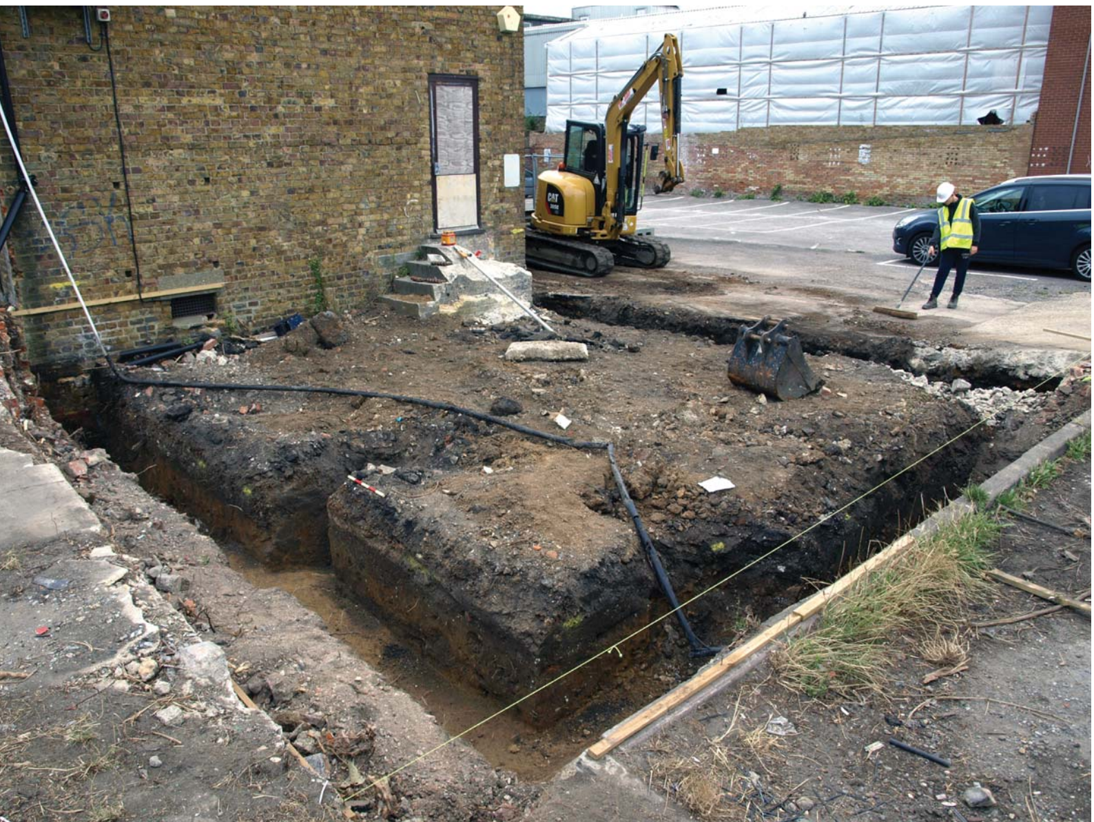
Plate 5: Looking north-east at foundations trench.
